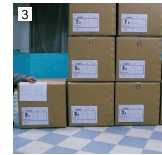
3 Correspond the general assembly drawing to the articles and find out the corresponding duct segments for installation
